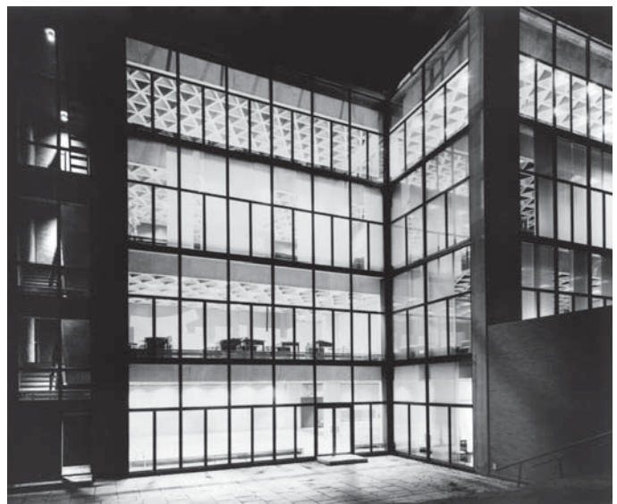
YUAG—Kahn Building, 1953. New window scrims control light, yet retain the building's translucency. When needed, blackout curtains offer total control of daylight.
